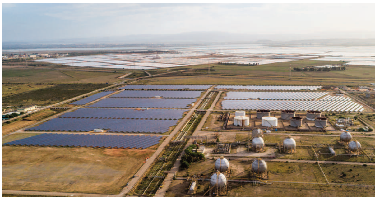
Assemini PV park, 23 MW. Cagliari, Italy.
