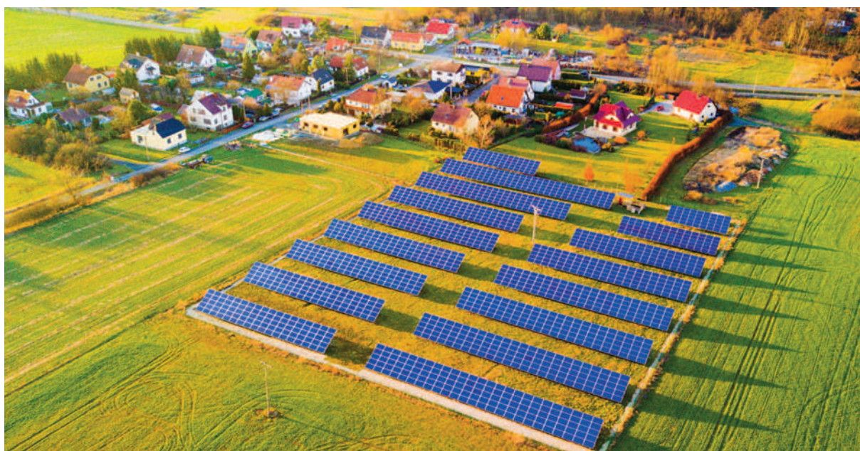
Ground-mounted PV park in Germany.
