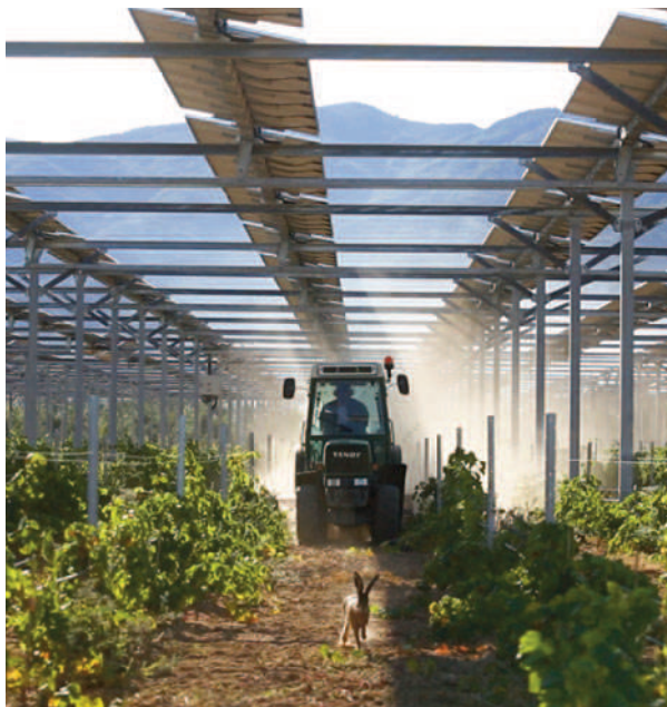
Dynamic shades Agri-PV system, viticulture.
