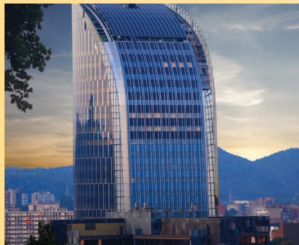
FINANCE TOWER, LIÈGE, BELGIUM, BIPV BY ISSOL, SIMCO ITALIA, JASPERS EYERS ARCHITECTS
