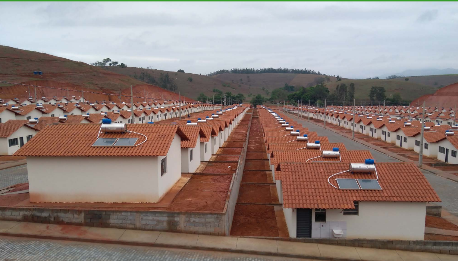
Around 400,000 thermosiphon systems were built in Brazil as part of the Minha Casa, Minha Vida social housing program.
