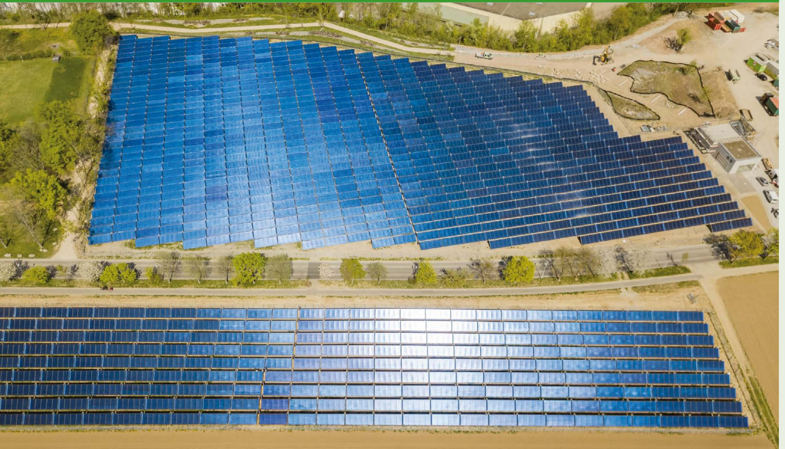
Germany's largest solar district heating system in Ludwigsburg with a capacity of 10 MW th was put into operation in early 2020.
