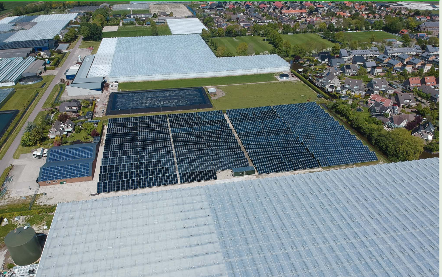
Collector system with 6.5 MW th for heating a greenhouse in Heerhugowaard, Netherlands. The application works as a drain-back system, which means that the collector fluid is water and not glycol.
