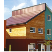
ÜserHuus AG (CH) NexPower Terra Cotta BIPV Thin Film Full Roof solution www.userhuus.ch
